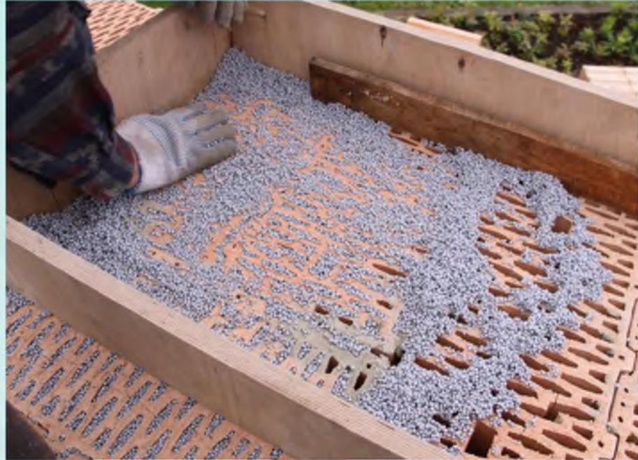
ceramic blocks with insulation material filling
