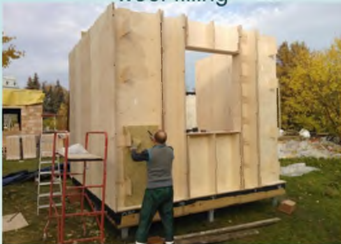
plywood frame with mineral wool filling
