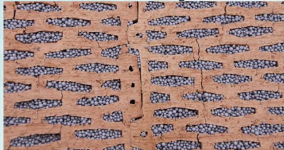
ceramic blocks with insulation material filling
