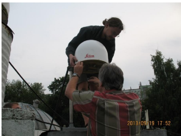
Picture 22. Calibrated Leica AR25 GNSS receiver antenna about to be installed at IGS/EUREF site Riga
